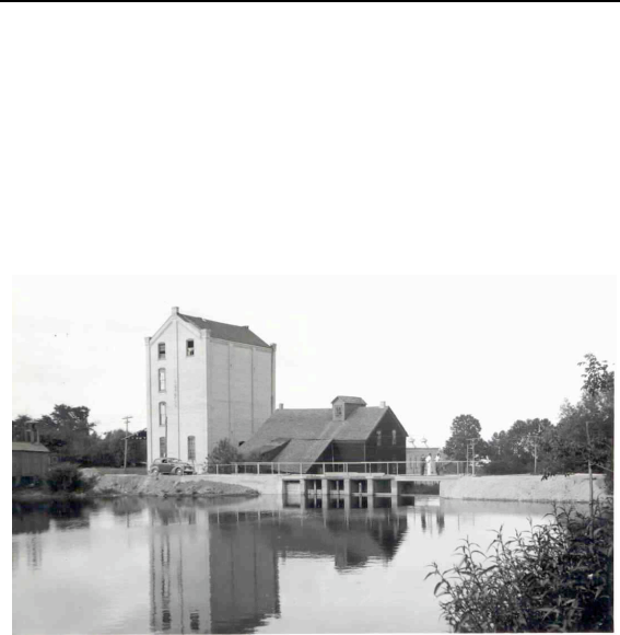
Reservoir Prior to Dam Removal
